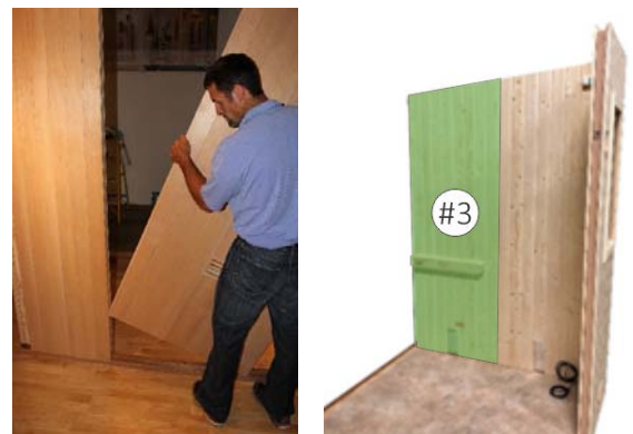
Figure 8. Installing Wall #3
