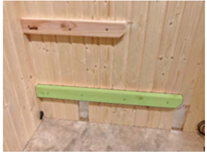
Figure 23. Installing Lower Bench Supports
