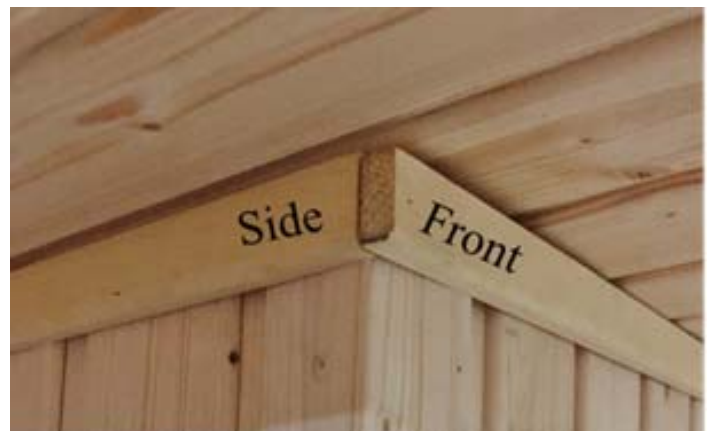
Figure 37. Installing Exterior Cove Trim
