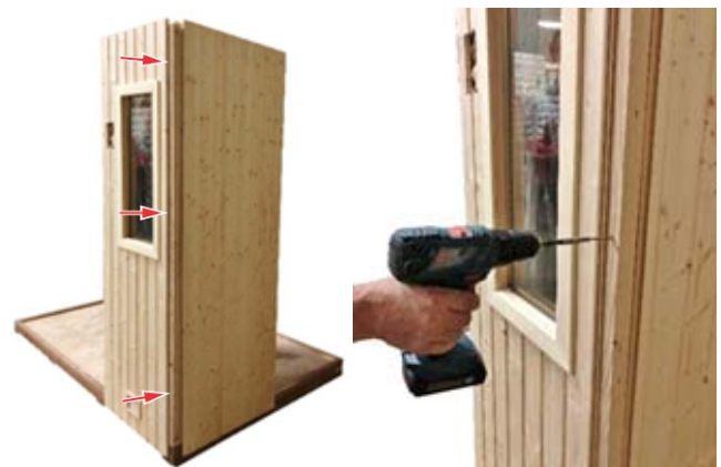
Figure 7. Attaching Wall #1 to Wall #2
