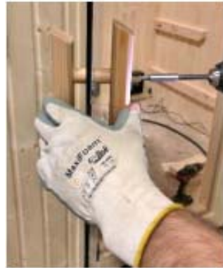
Figure 18. Installing Door Handle
