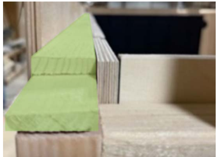
Figure 19. Installing Back Top Plate
