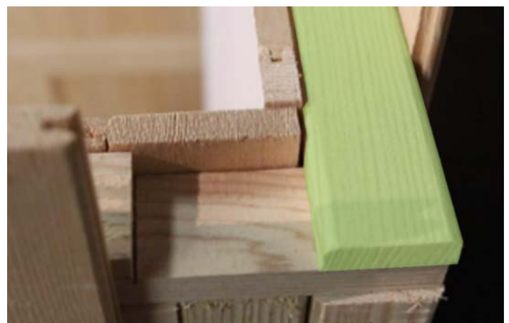
Figure 20. Installing Left Top Plate
