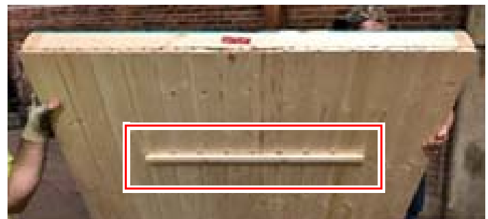
Figure 30. Placing the Right Roof Panel
