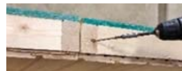
Figure 31. Toe Nailing Roof Panels Together
