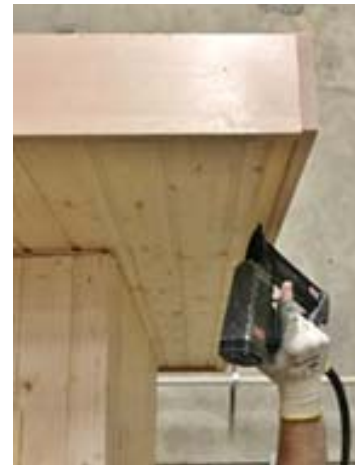
Figure 36. Installing Soffit Trim
