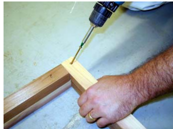
Figure 3. Laying the Base Rail
