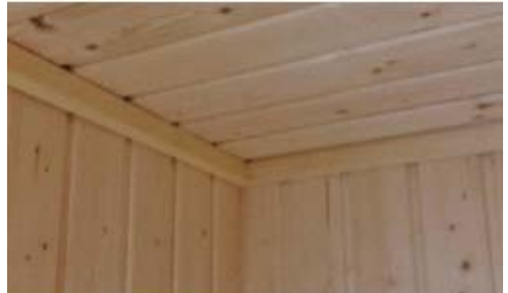
Figure 38. Installing Interior Cove Trim
