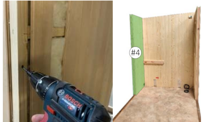
Figure 10. Installing Wall #4
