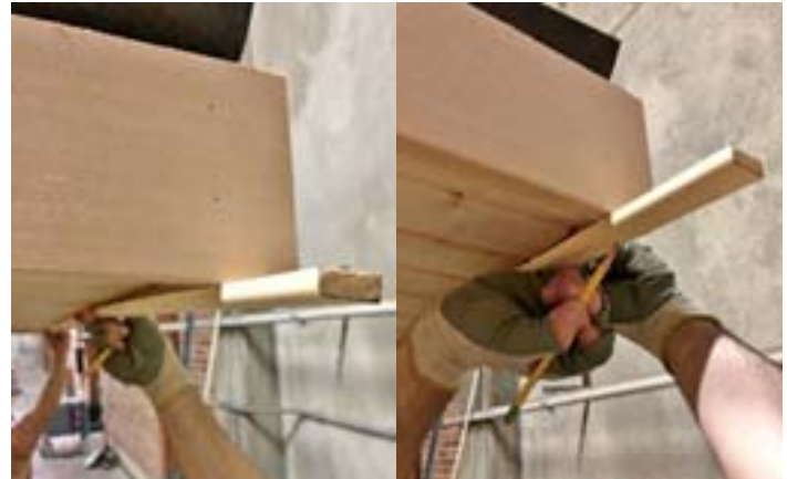
Figure 35. Measure, Mark, and Cut Soffit Trim
