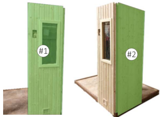
Figure 6. Installing Walls #1 and #2
