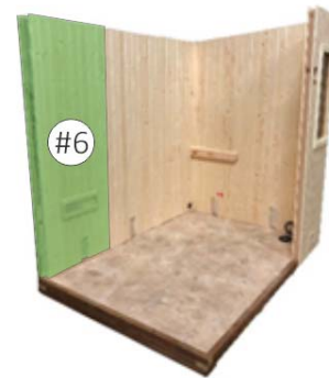
Figure 12. Installing Wall #6
