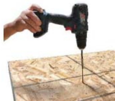
Figure 32. Attaching the Roof
