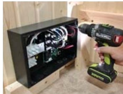
Figure 25. Attaching the CB Box
