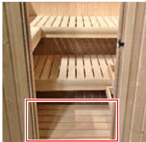
Figure 43. Placing Duck Board
