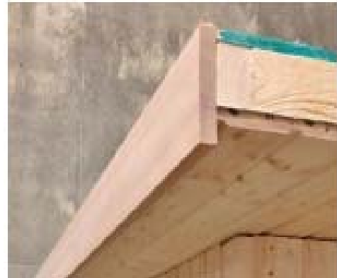
Figure 33. Installing Back Wood Fascia
