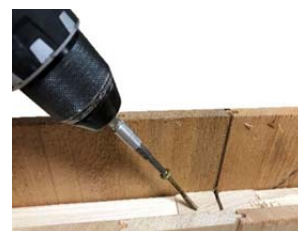
Figure 9. Toe-Nailing Example
