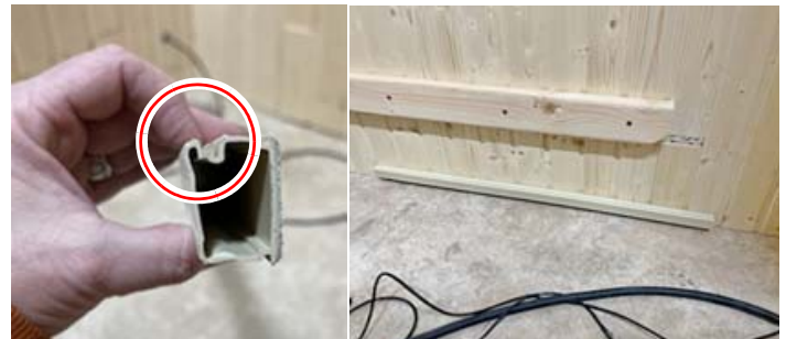
Figure 26. Orienting and Installing Cable Track
