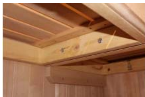
Figure 42. Attaching Return Bench to Upper Bench
