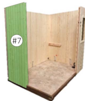
Figure 13. Installing Wall #7
