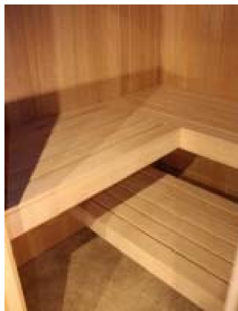
Figure 41. Installing Return Bench
