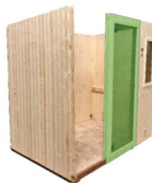
Figure 15. Installing Door Panel Assembly
