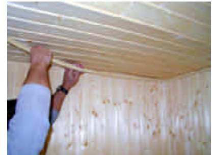
positioning cove molding
