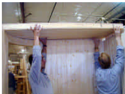
placing ceiling panel A into position
