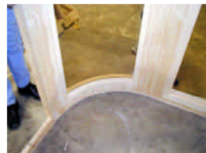
panel 9 positioned on base rail
