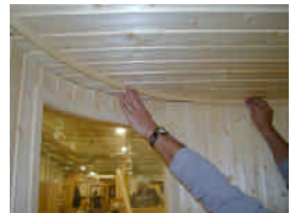
flexing the cove molding
