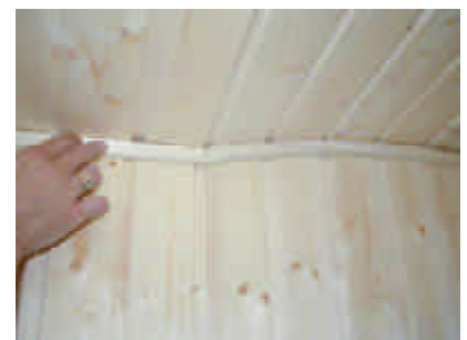
finished cove molding
