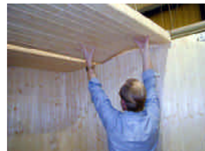
placing curved ceiling panel B into position
