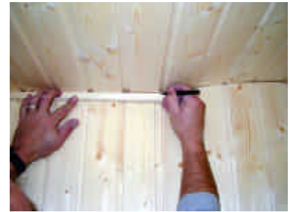
marking cove molding
