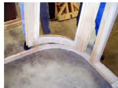
placing panel 9 on base rail
